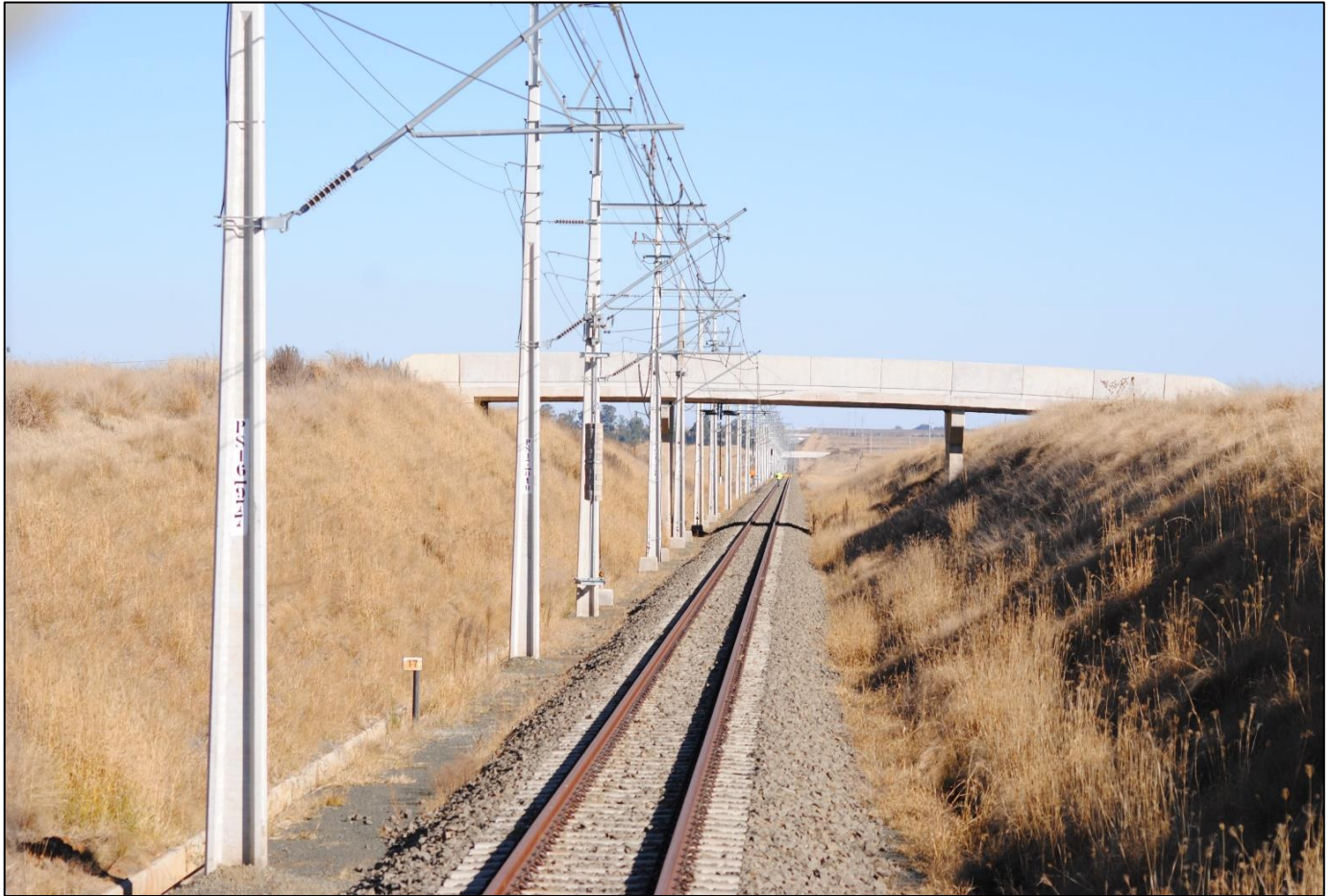
25kV AC AUTO-TENSIONED OHTE - MAJUBA RAIL ELECTRIFICATION PROJECT
